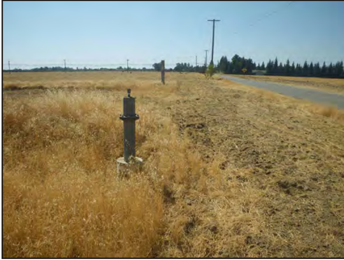
Photo 1 – View west along GWD 12/14-inch pipeline alignment that traverses the northern portion of the project site. International Avenue at right.
