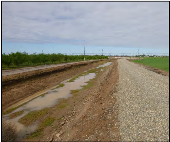
Photo 4. View W along the Enterprise Canal at the southern edge of the project area.
