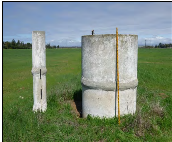
Photo 4. Concrete irrigation stand pipes (Feature 5), facing N.
