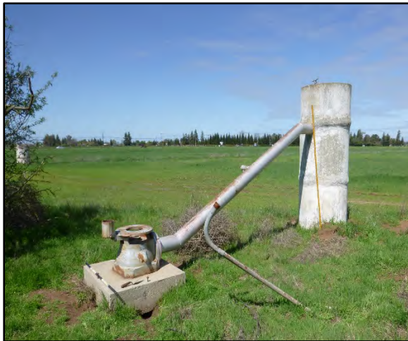
Photo 3. Well head and stand pipe (Feature 4), facing NW.
