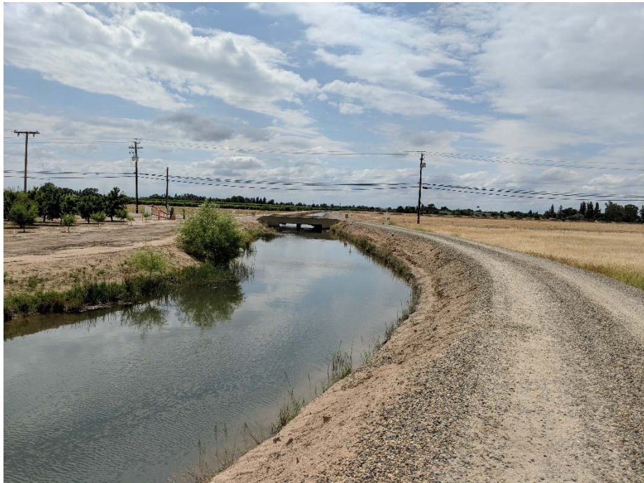
Enterprise Canal and Minnewawa bridge with cliff swallow nesting colony on adjacent land to south of project area. Looking west.
